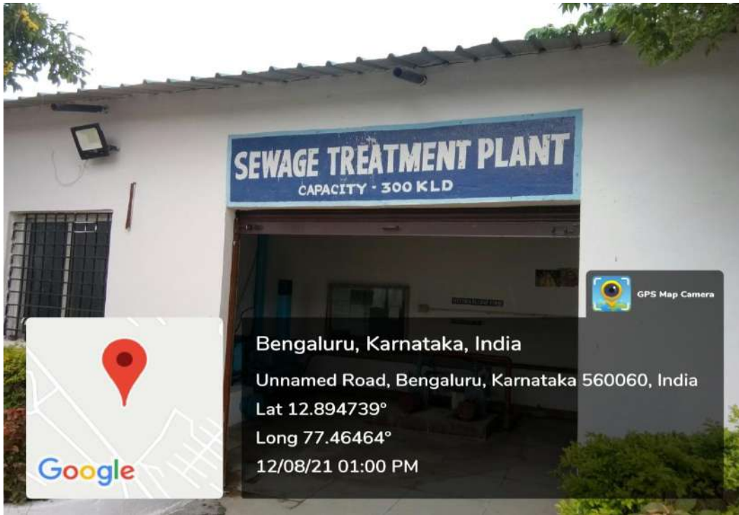
Photo: Sewage Treatment Plant
