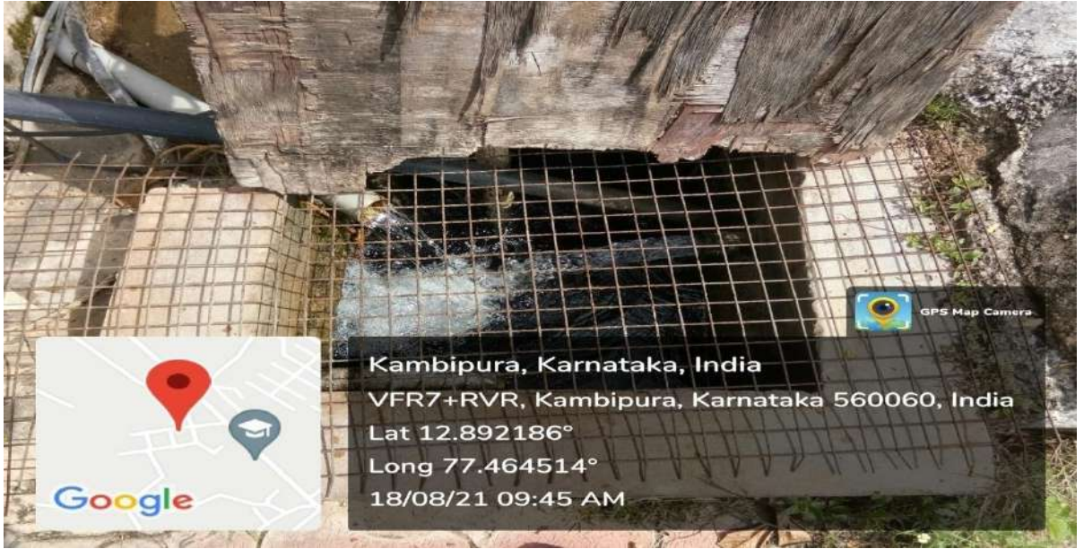
Photo: Underground water Storage Tank in the Campus
