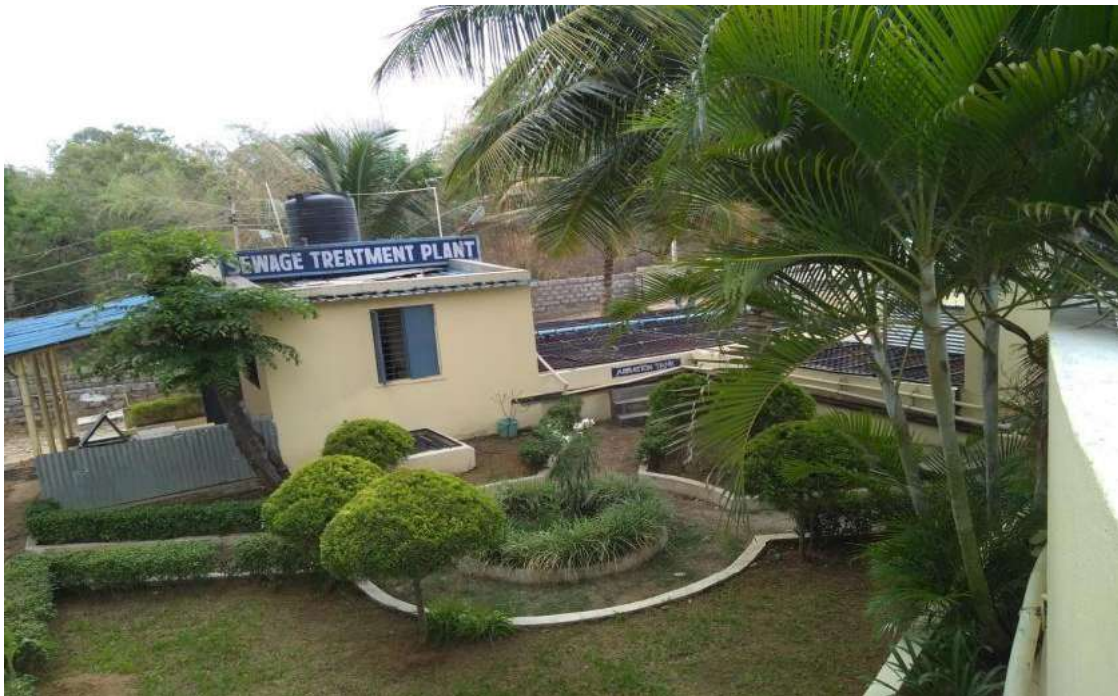
Photo: Sewage Treatment Plant (250 KLD)
